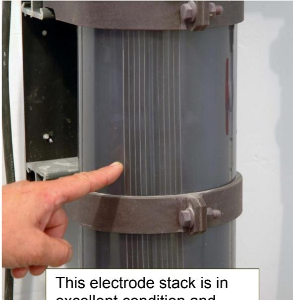
This electrode stack is in excellent condition and does not require cleaning
